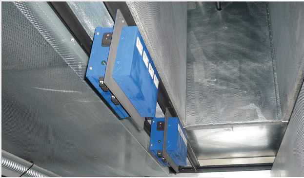
Plasma Air's needlepoint bipolar ionization equipment was easily installed in the facility's air handling units.
