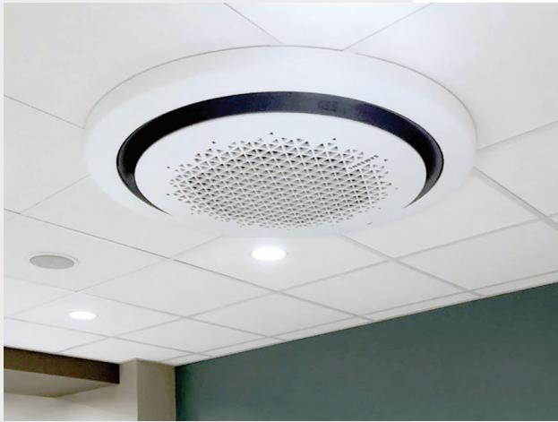
Plasma Air model PA664 was installed in multiple VRF round cassettes and ducted air handling units.
