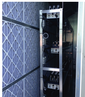
Slide-in rack installation for mounting of the ionizers in any air handler.
