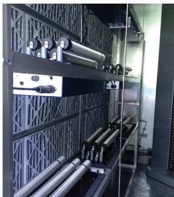
Slide-in rack installation for mounting of the ionizers in any air handler.
