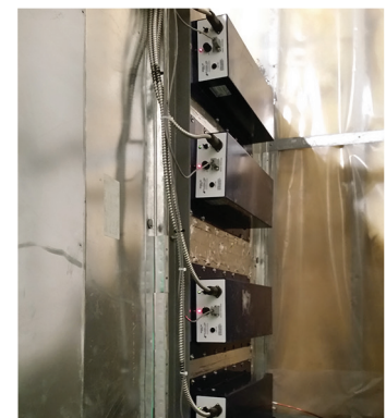
Ionizers mounted around the perimeter of a supply duct.
