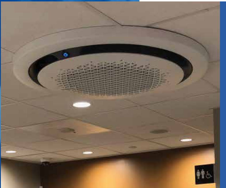
Plasma Air model PA664 was installed in multiple VRF round cassettes and ducted air handling units.
